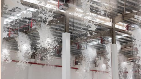
Fire-fighting Hi-Ex Foam System for DG
